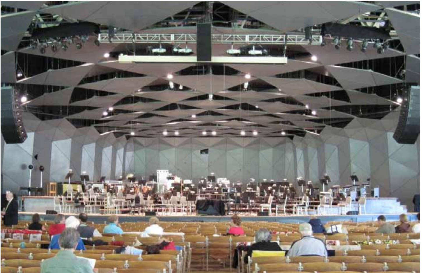
Figure 2: Overhead panels at the Shed at Tanglewood, Lenox, MA.
