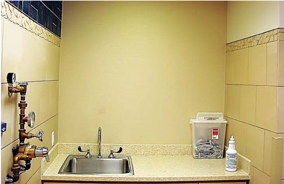
Fig. 2. View of the acoustically absorptive treatment in the remodel of a burn acute care unit. An absorptive panel is wall mounted behind the sink in the interior of a debridement treatment room (Reprinted with permission from ref. 46. Copyright 2008, Institute of Noise Control Engineering).
