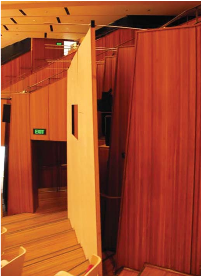
Fig. 6. One of the adjustable medium density fiberboard (MDF) panels covering the lower sawtooth walls during the 2009 acoustics trials in the Concert Hall at the Sydney Opera House.
