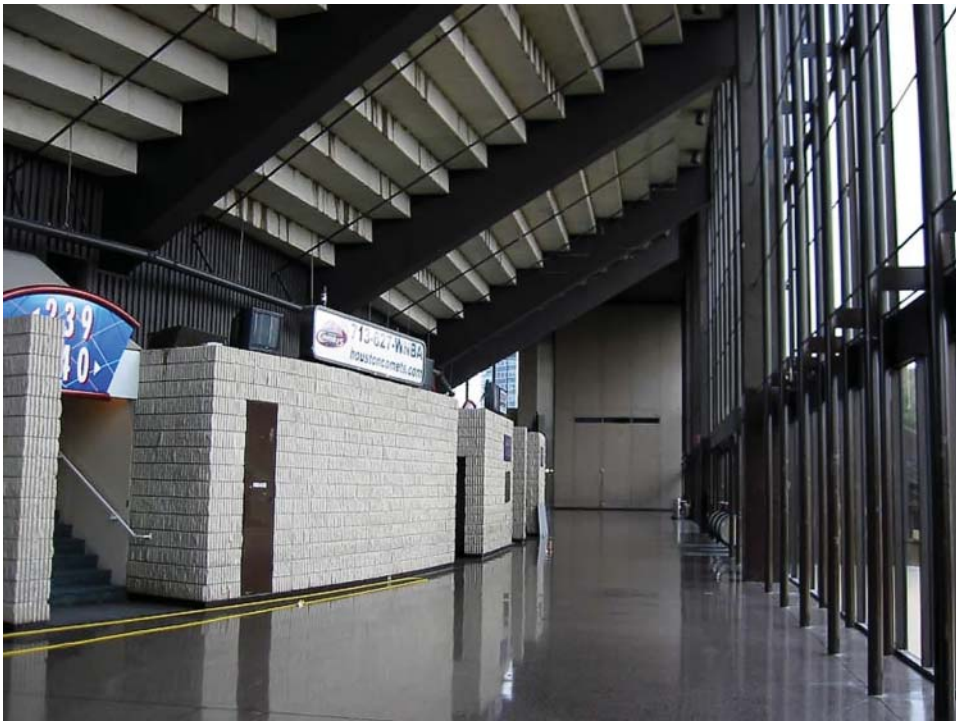
Fig. 2. High background noise levels at the Lobby Level can be traced to the use of hard, reflective surfaces including the terrazzo floor, the glass curtain walls, and the exposed concrete seating structure. Sound isolation was poor at the south side of the Lobby where traffic noise was transmitted through the glass curtain wall. This was the main cause for the high background noise levels.
