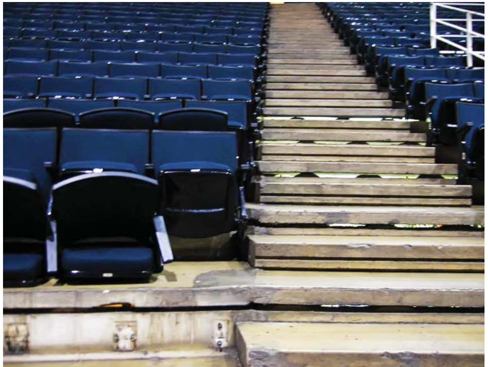
Fig. 3. Seating in the Compaq Center consists of upholstered fabric seats and backs that are useful in decreasing midfrequency reverberation times to suitable lengths. Many large ventilation slots are visible in the concrete seating structure and contribute to poor sound isolation between the main bowl and the Lobby Level.
