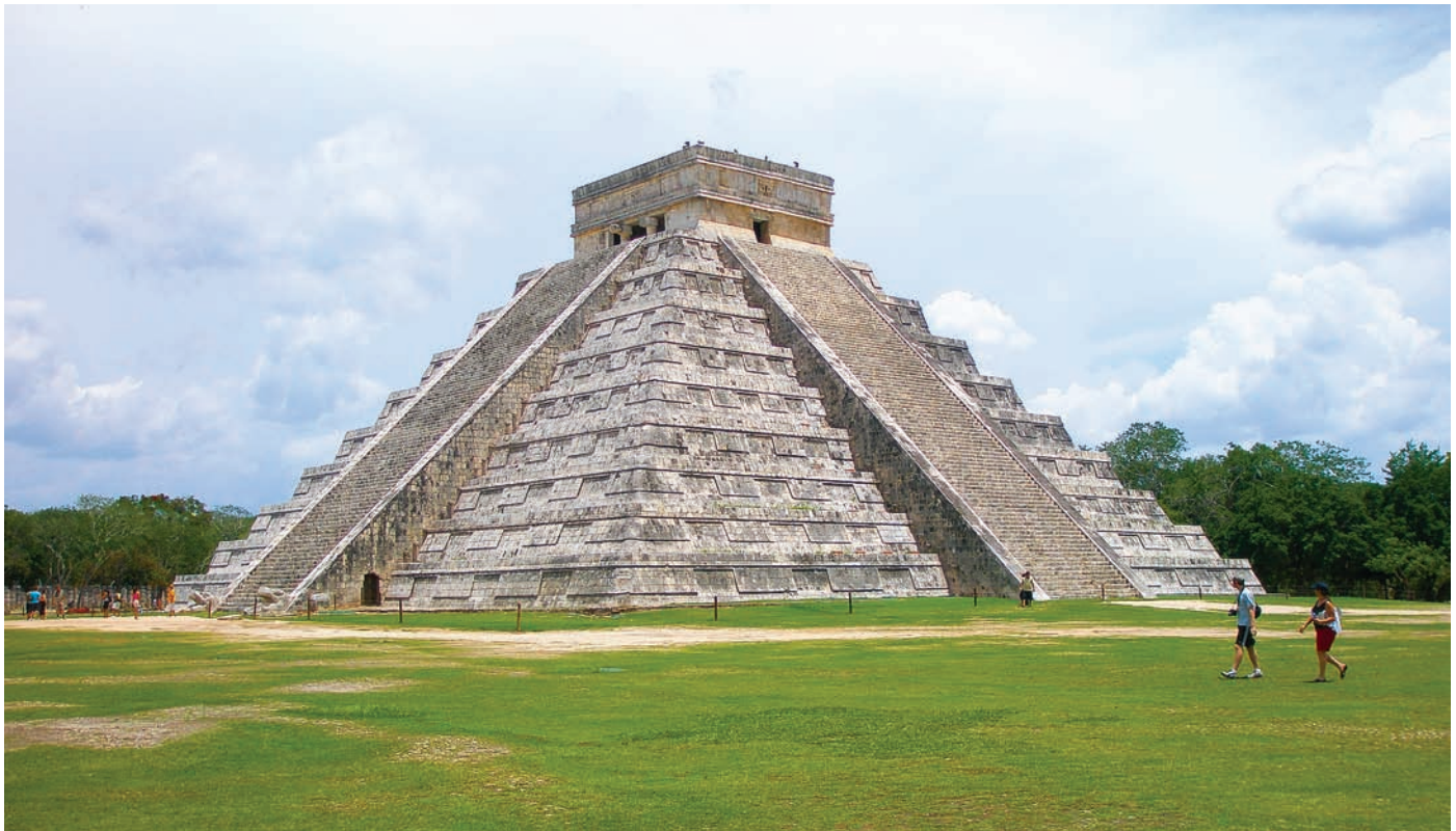
Fig. 6. The El Castillo pyramid of Chichen Itza (photo taken by the author).
