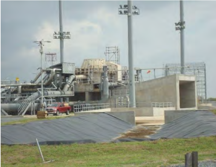
Figure 4. The Antares launch pad at the Wallops Flight Facility, Virginia. The rocket is attached to the pad by the rocket launch mount, which is the large white ring that can be seen in the middle of the figure. The (square) rocket flame trench exit is shown at right .
