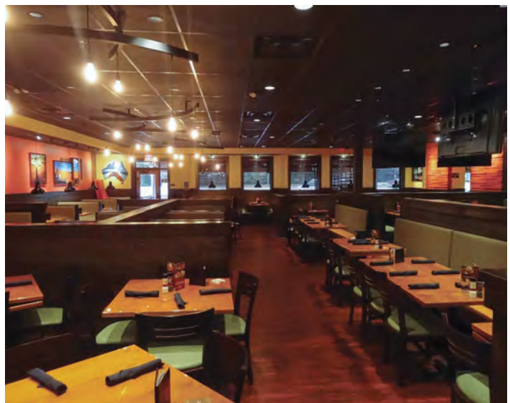
Figure 2. All of these restaurants suffered from acoustic defects and all having a varying amount of absorbing material. Top: Heavy carpet, drapery, and upholstered seating. Center: Mainly reflective materials. Bottom: Acoustic ceiling tile (in grid).
