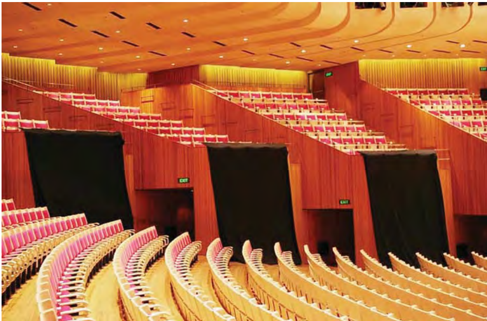
Fig. 5. Fabric panels in place over the lower “sawtooth” walls in the Concert Hall at the Sydney Opera House.
