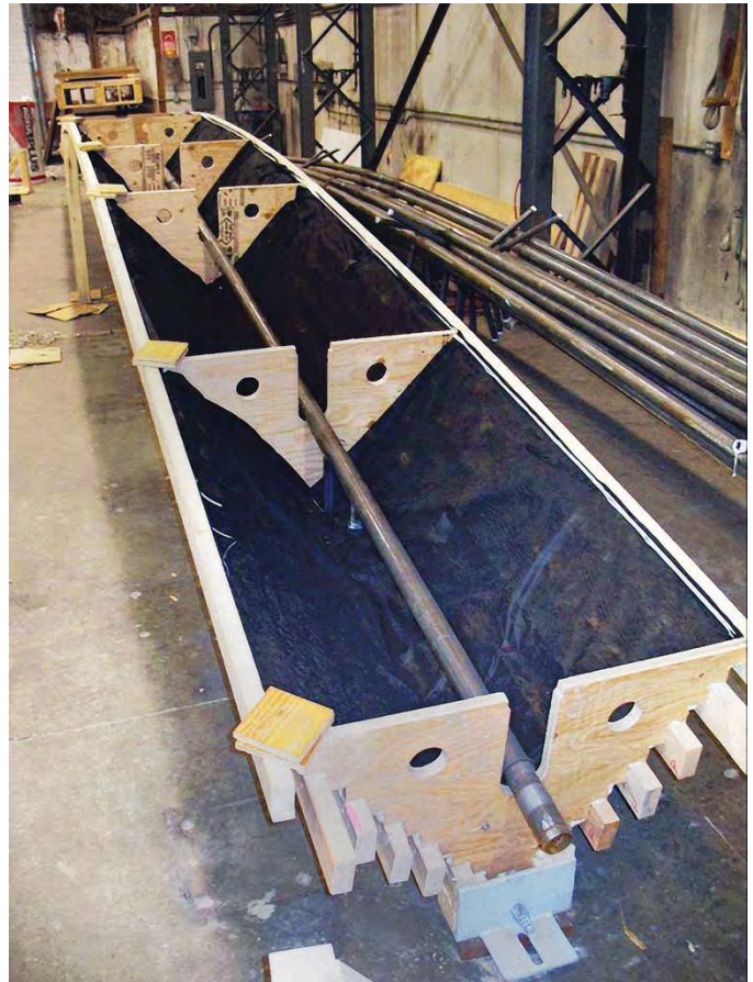
Fig. 5. Interior of vee-shaped WoodWave© structure during construction (Courtesy StructureCraft Builders).
