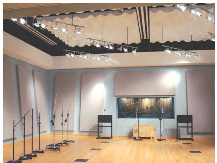
Fig 12. (top) An optimized curved surface designed to be tiled in a modulated array. (bottom) Ceiling Waveform treatment at KTSU, Houston, TX. (Photo Courtesy of HFP Acoustical Consultants)
