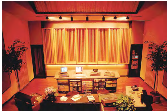
Fig 7. Gateway Mastering, Portland, ME showing a fractal diffusing rear wall (Diffractal ® ). (Photo courtesy of Gateway Mastering & DVD).
