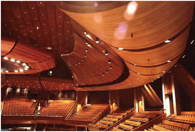
Fig 5. Schroeder diffusers in the Michael Fowler Centre, New Zealand. (Photo courtesy of Dr. Harold Marshall of Marshall Day Acoustics)
