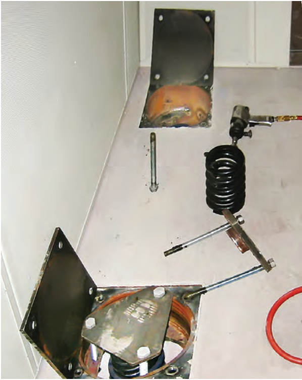
Fig. 2. Spring isolators during installation.
