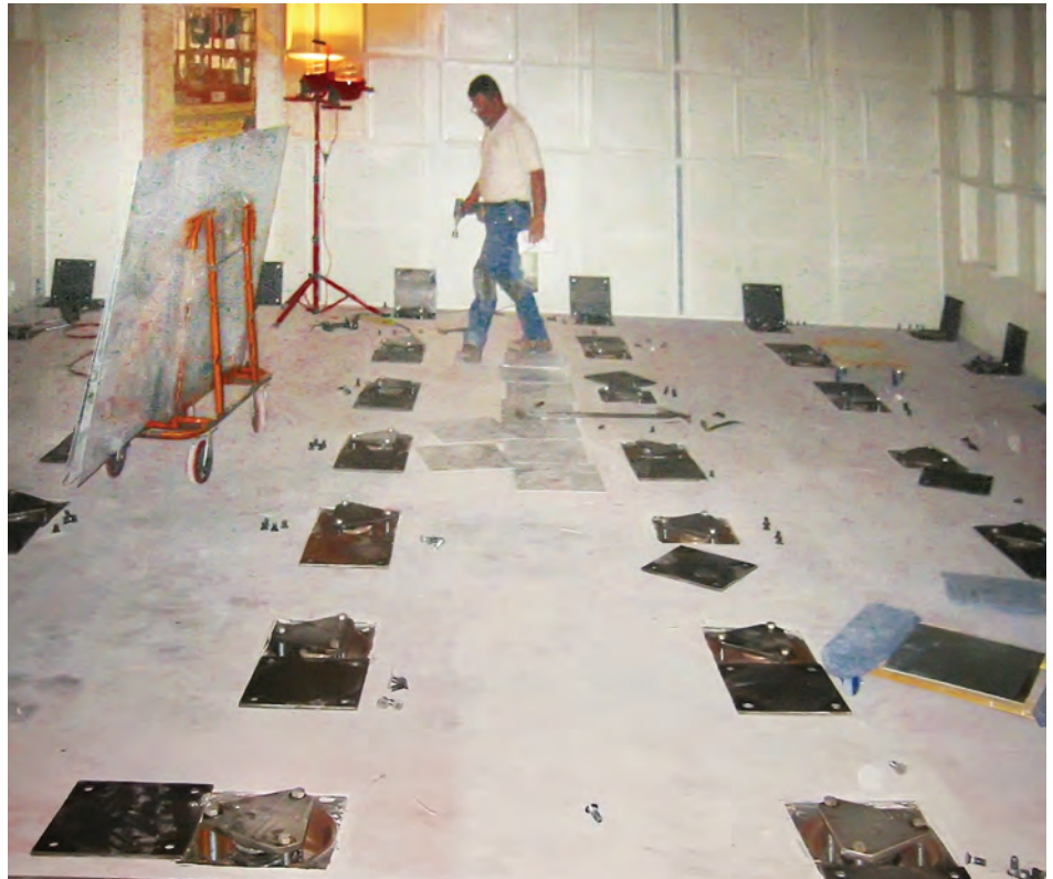
Fig. 3. Raising the inner chamber.
