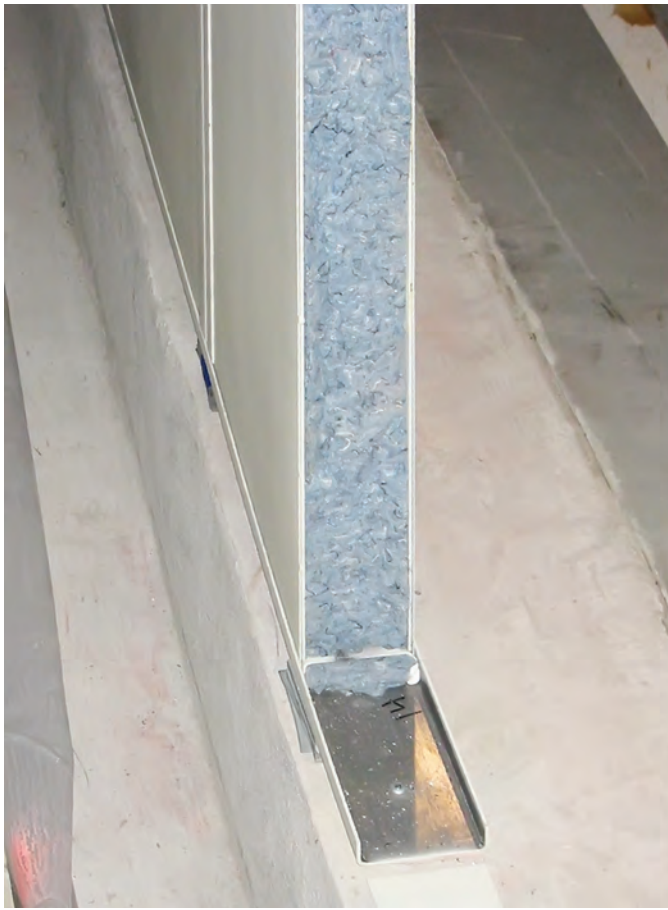
Fig. 4. Outer chamber wall install in a perimeter channel.
