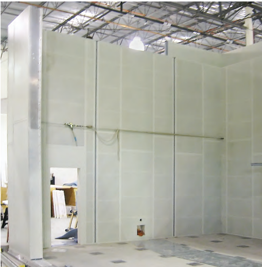
Fig. 5. Inner and outer chamber walls during construction.
