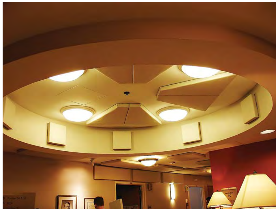
Fig. 3. View of the acoustically absorptive treatment in the remodel of a hematological cancer unit. Sound absorbing panels are mounted high on the walls and on the ceiling of the corridor, as well as in the large circular architectural feature at the nurses' station. Note a person shown at the bottom center for scale (Reprinted with permission from ref. 30. Copyright 2007, Acoustical Society of America).
