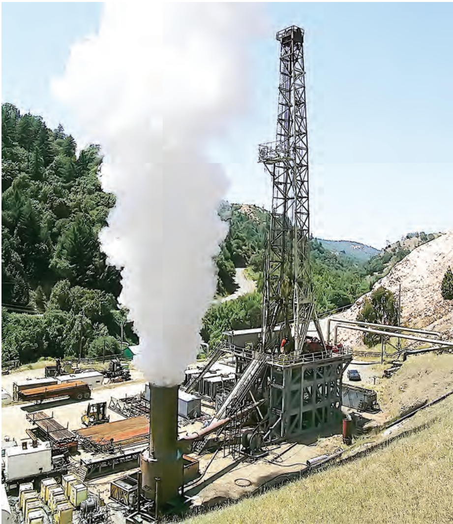
Fig. 2. Drilling a steam well at the Geysers (Courtesy Calpine Corporation).
